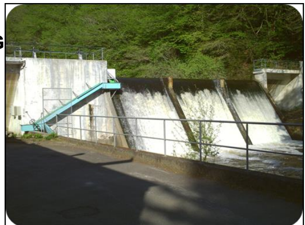
The prefabricated crawling gutter with two resting pool.
