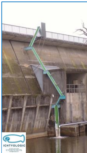
Dam of Rochereau, Lay River \Delta h = 11.00 m
